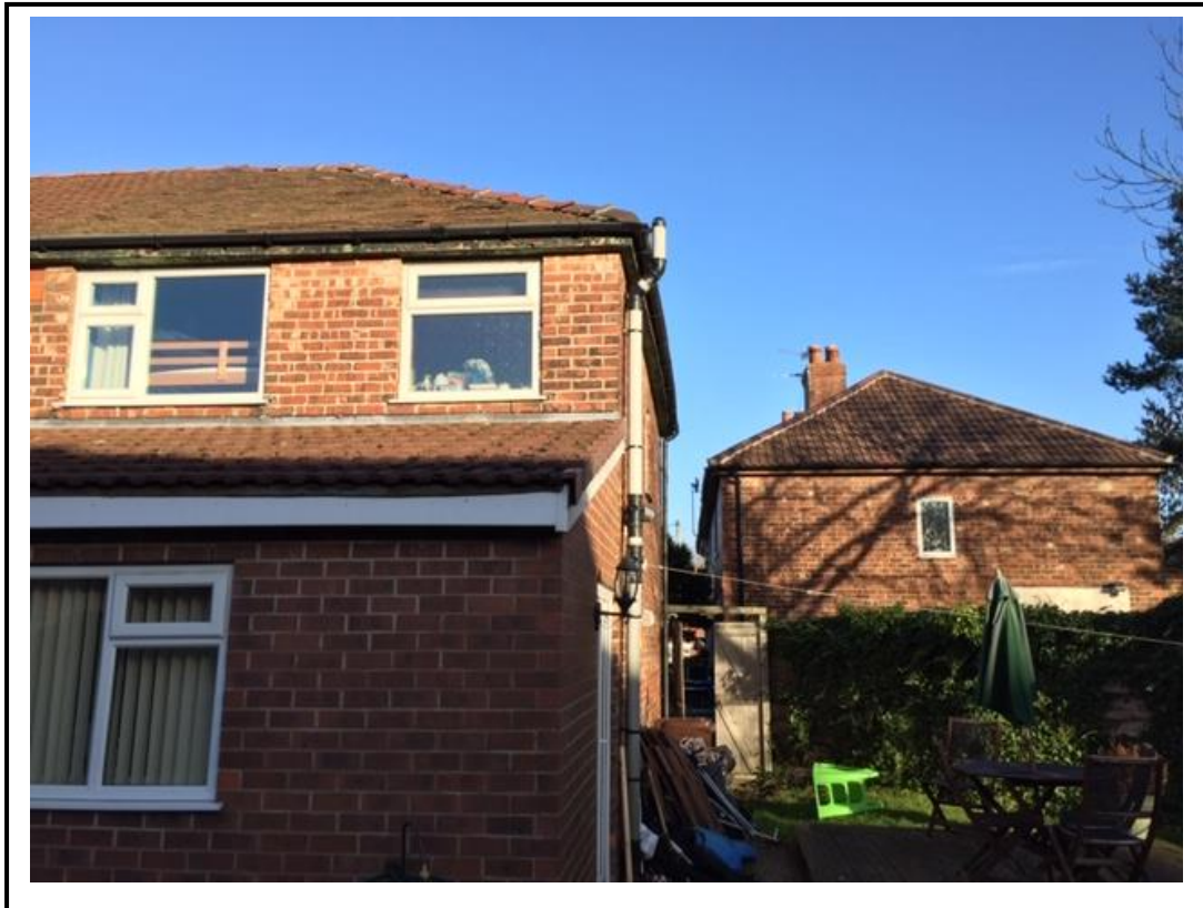
Photo 3 – view of common boundary between no. 5 and no. 4 Bankfield Avenue
