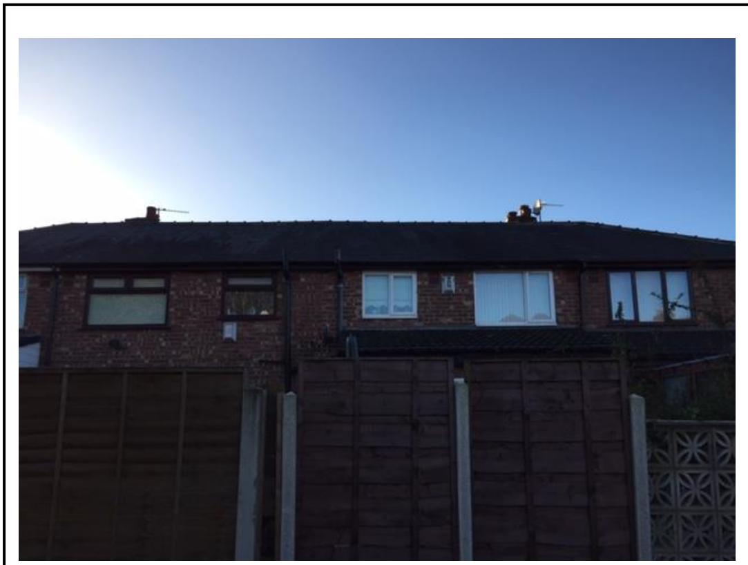
Photo 4 – view of the rear elevations of the properties at 34-40 Sunnyside Road to the rear of the site
